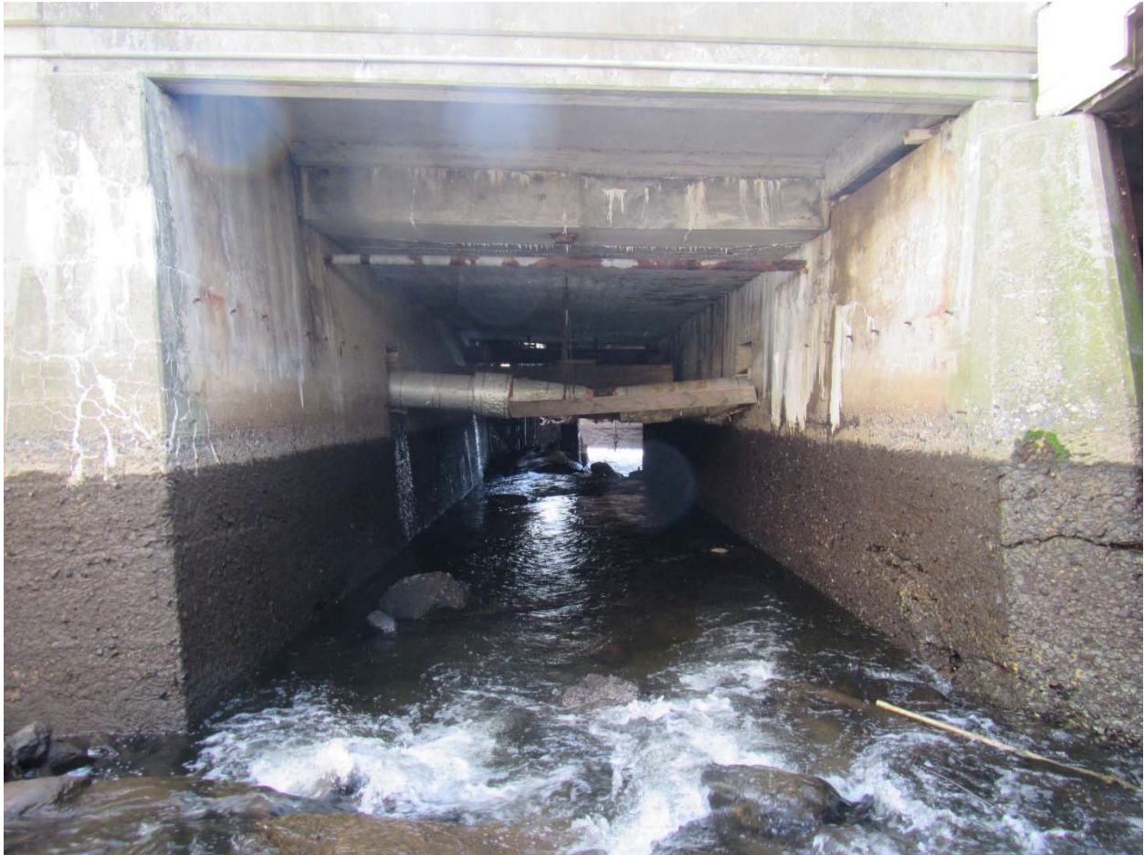
Figure 25. View downstream through north span of Main Street bridge in drawn down condition, May 8, 2018. Stain lines indicate normal pool elevation.
