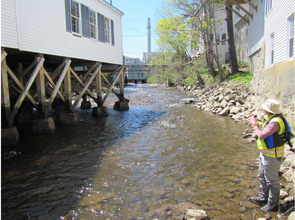
Figure 27. Looking upstream from Main Street with impoundment drawn down, May 8, 2018. In addition to infrastructure in the river, natural features such as boulders, mid-channel bars, riffles, and pools are all present through this reach.
