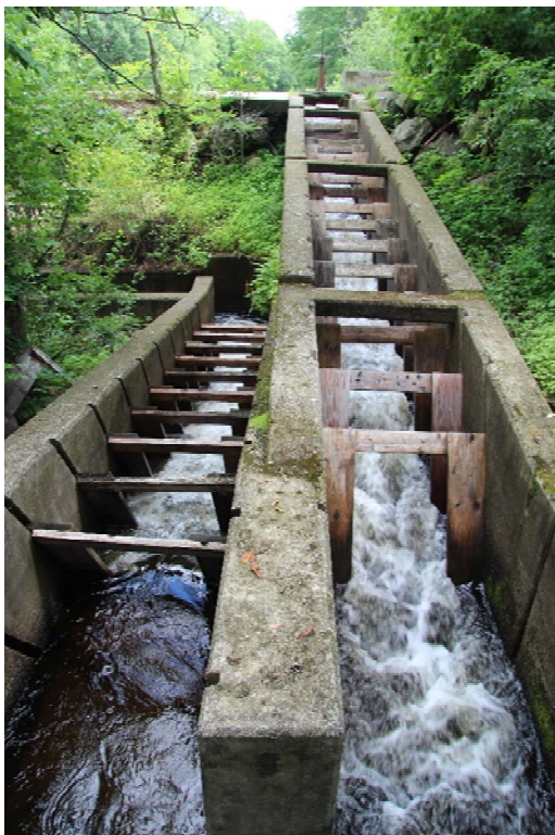
Figure 46. Example of a Denil fishway.
