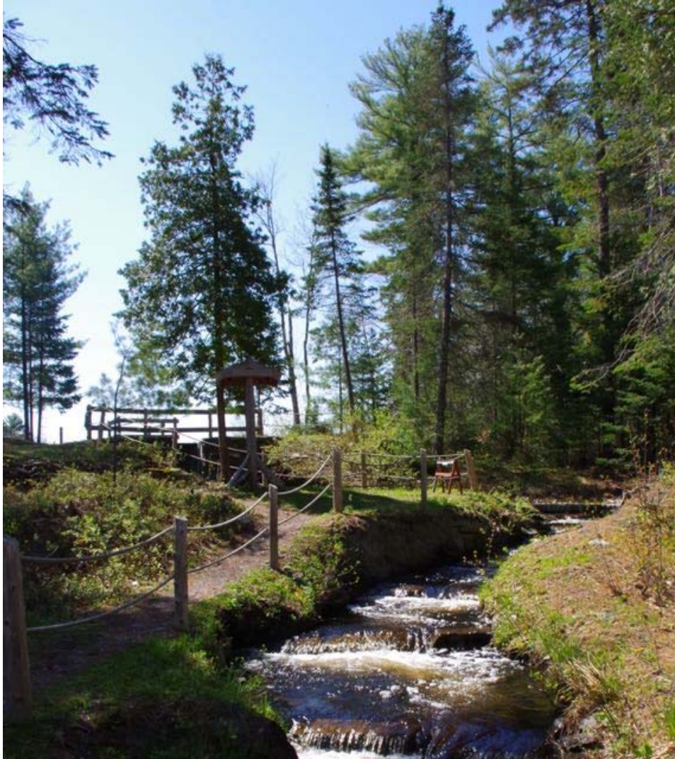
Figure 45. Pool and weir fishway at Blackman Stream (photo credit: Maine Sea Grant).
