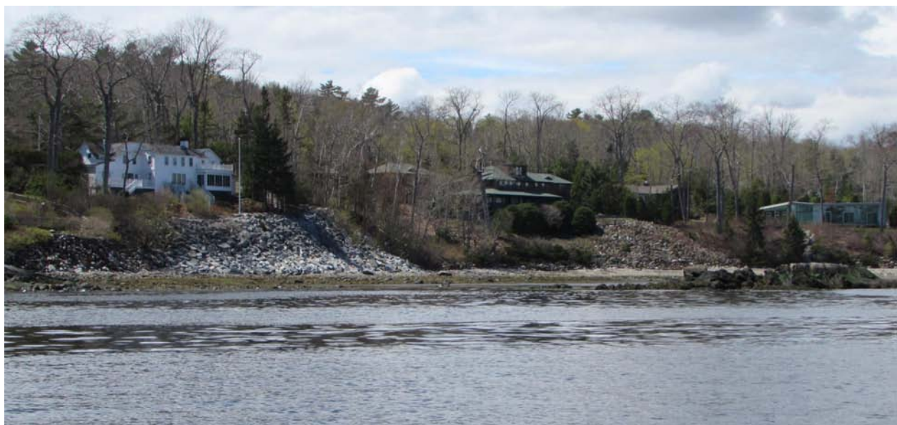
Eroding and hardened bluffs south of Dillingham Point
