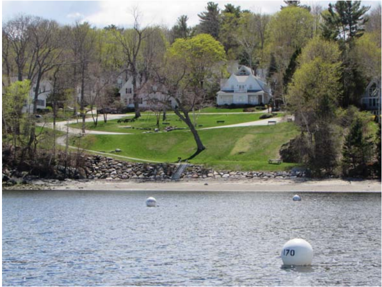
Laite Beach with rock work in places to protect shore from erosion
